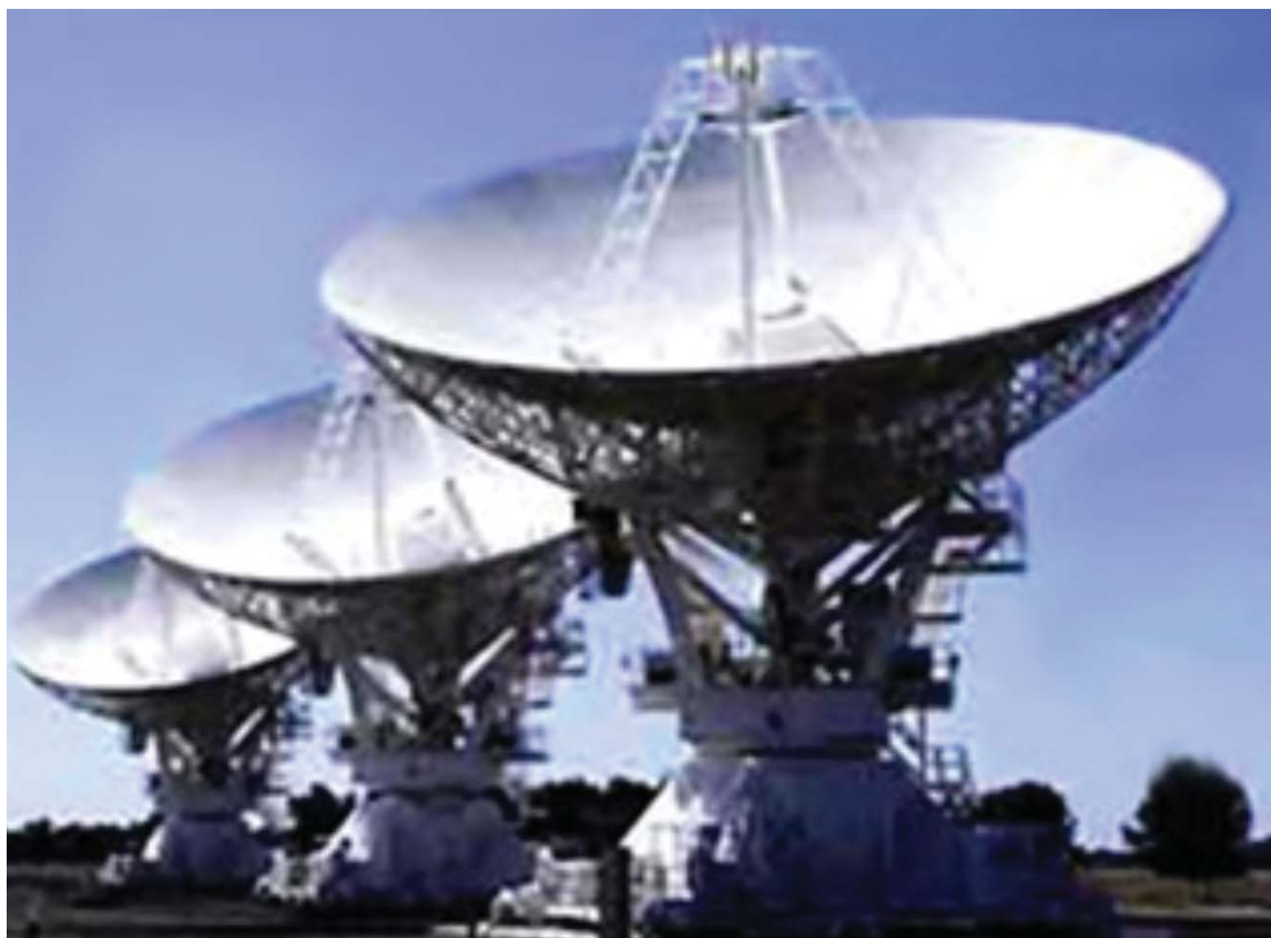
Satellite Earth Station
