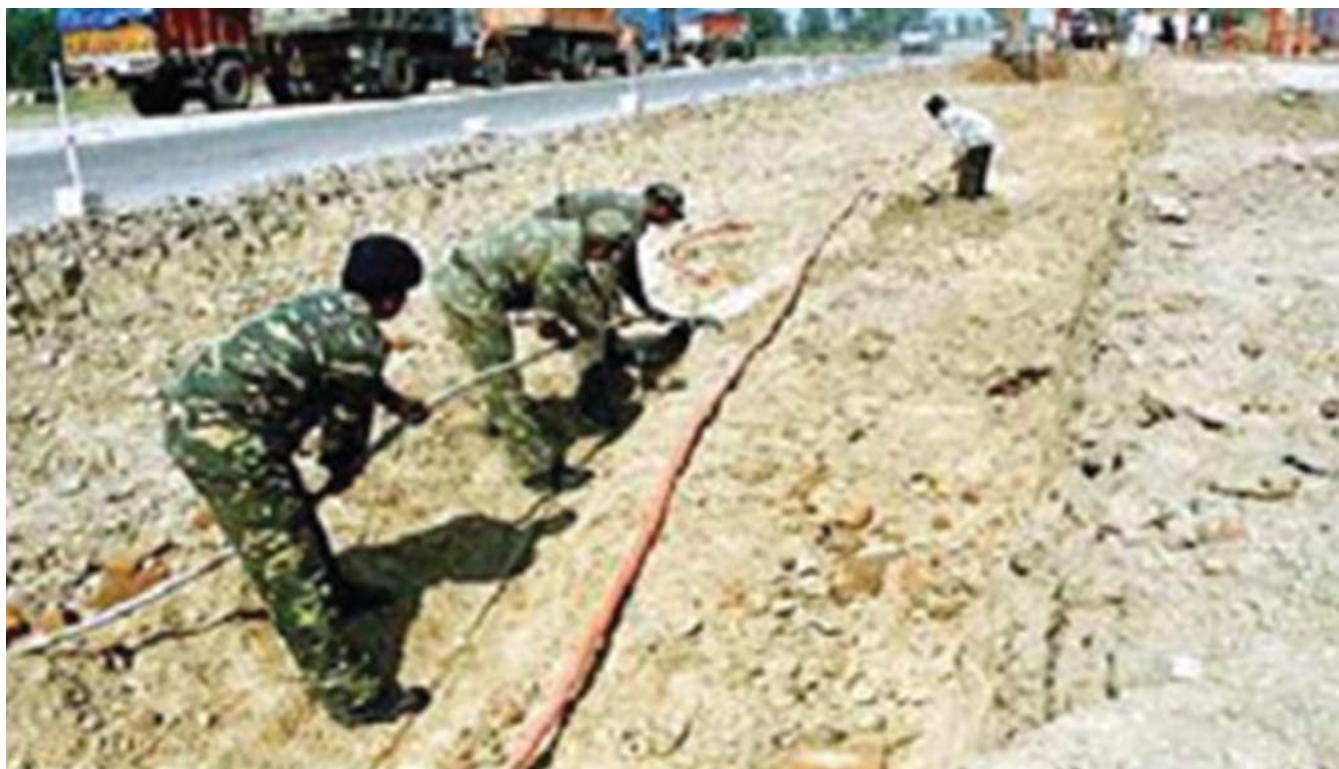
Telephone cable laying Work-in-Progress
