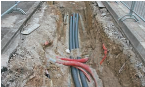
Trenching work for laying Optical Fibre Cable under progress
